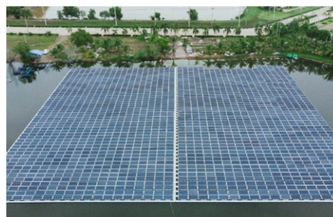
Picture showing the solar power plant project, installed on the water at Prachinburi Glass Industry Co., Ltd., size 696.80 kW.
