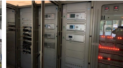
Picture depicts Microgrid controller of Microgrid Development Project at Mae Sariang District, Mae Hong Son Province, of the Provincial Electricity Authority.
