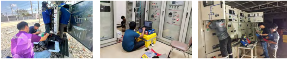
The image showing the Testing and Commissioning at substation
