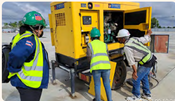
Site Safety Inspection
