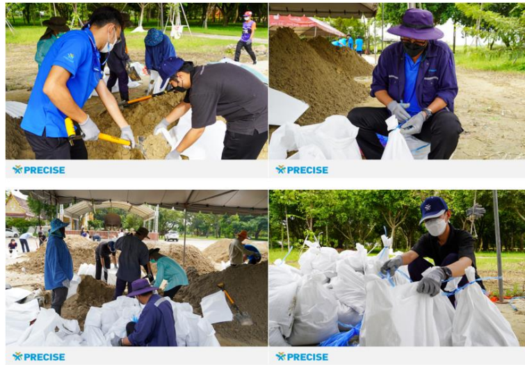
October 5, 2022: The first sandbag filling
