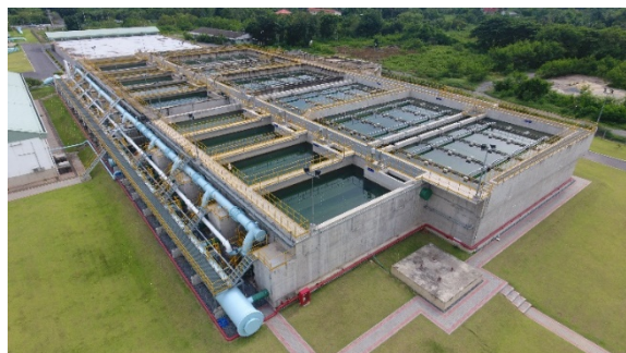
Samkhok Water Treatment Plant (formerly name Pathumthani Water Treatment Plant)
