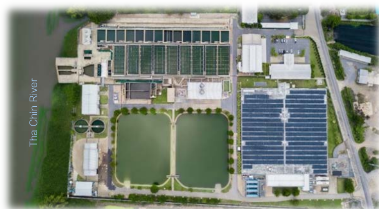
Banglen Water Treatment Plant
