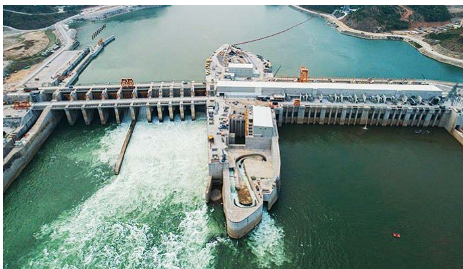
Xayaburi Hydroelectric Power Project, Lao PDR, of Xayaburi Power Co., Ltd., one of the businesses invested by CKP.
