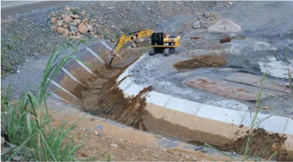
(above) Photographs of construction of open drain in the water drainage management within the Project
