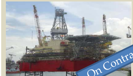
AOD III Jack-up Rig*
