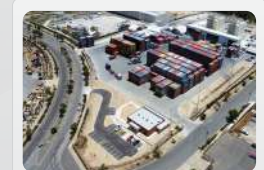
Hope Valley Distribution Center
