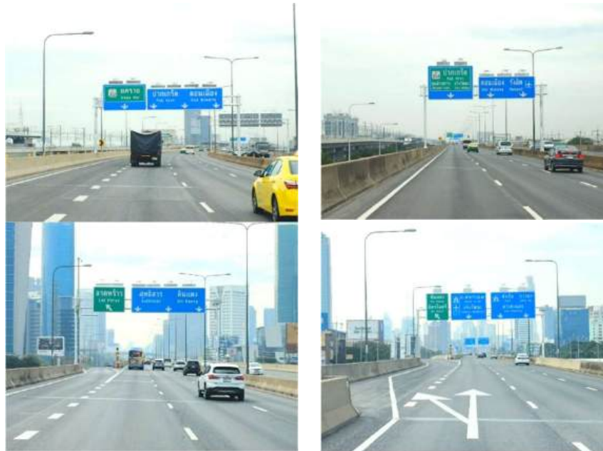
Improvement of traffic signs on the elevated road
