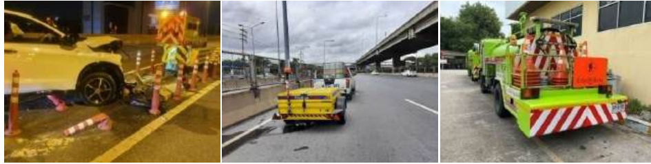
Actions taken to reduce severity of accidents: installments of crash cushions and truck mounted attenuators
